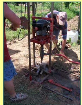
Ray and Gene adding a drill shaft to drill deeper
